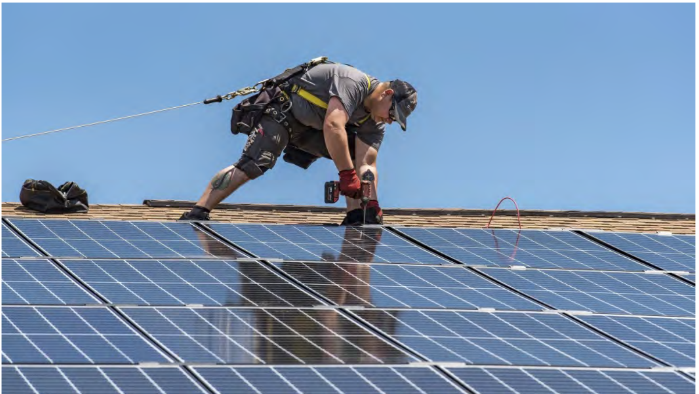
Installing solar PV panels on a home in the Dover Air Force Base in Delaware. Credit: Roland Balik, U.S. Air Force.
