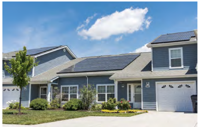
Rooftop solar panels at the Dover Family Housing Community. Credit: Roland Balik via United States Air Force, CC BY 1.0.
